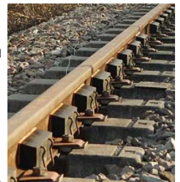
Clip on Corus rail dampers attached to an SNCF track.
